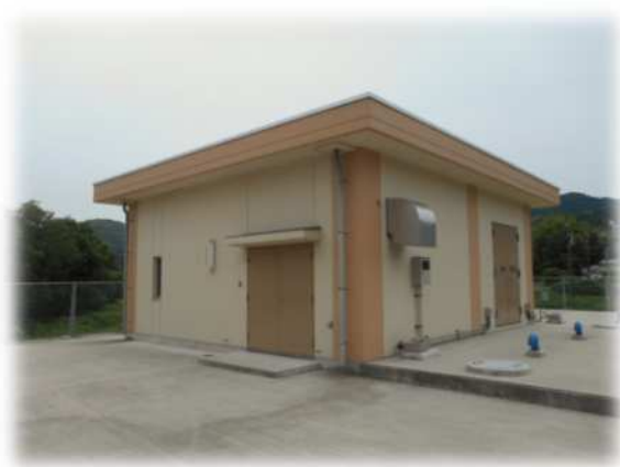
[ポンプ場（熊毛送水）]
