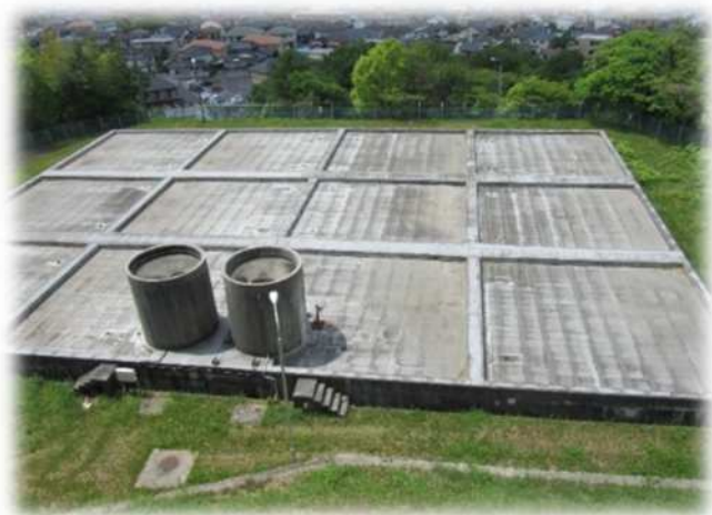
[大迫田低地区配水池]
