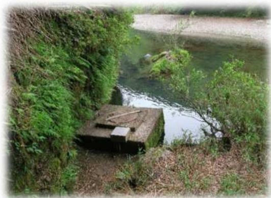
[取水場（錦川表流水）]
