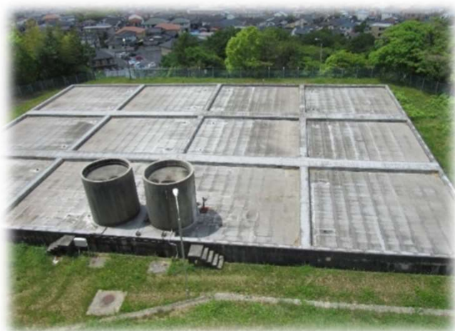
[大迫田低地区配水池]
