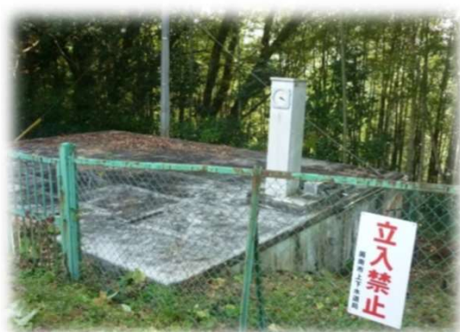
[須万市配水池]
